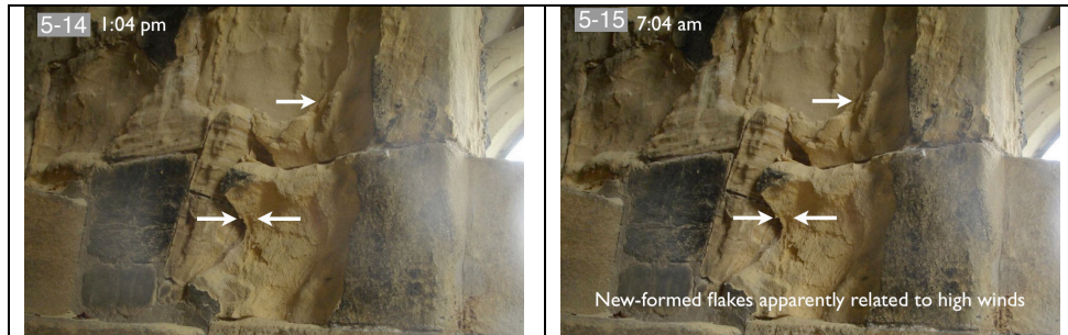
Figure 6. Two time-lapse images showing the episodic loss event seven days later than in Figure 5 with new losses taking place at white arrows (May 15, 2007).
