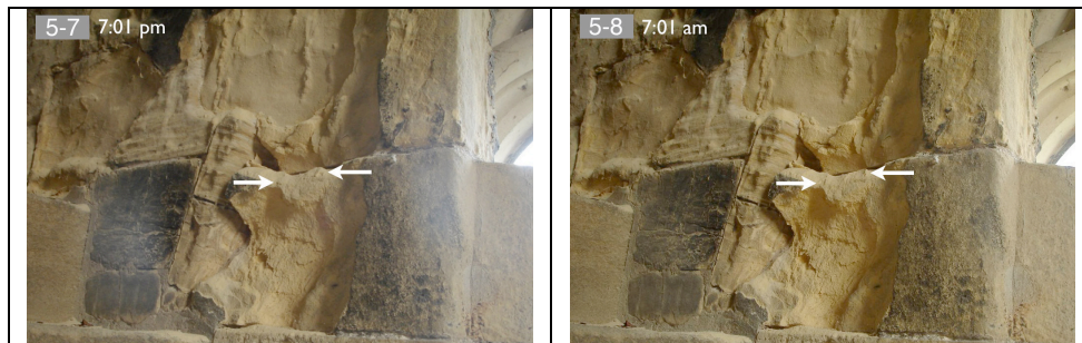
Figure 5. Two time-lapse images showing an episodic loss event on May 8, 2006 with loss of stone surface taking place at white arrows.
